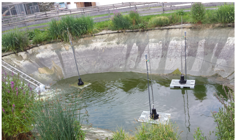
Infuses oxygen and prevents biological stagnation of water: Submersible aerator TRN by Tsurumi, here are three small devices that stand freely on the base of the tank – the water has been pumped out for simultaneous restoration of the tank
