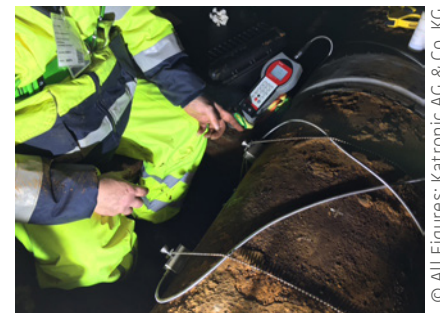
Figure 3: Engineer using a portable KATflow 200 ultrasonic flowmeter to obtain provisional flow data
