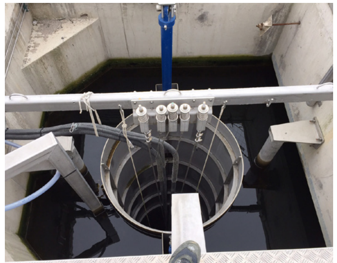
Each of the machines was built into a pipe barrel
