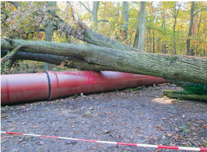
Figure 8: An uprooted oak tree which fell onto the interim pipeline did not result in any operational disruptions
