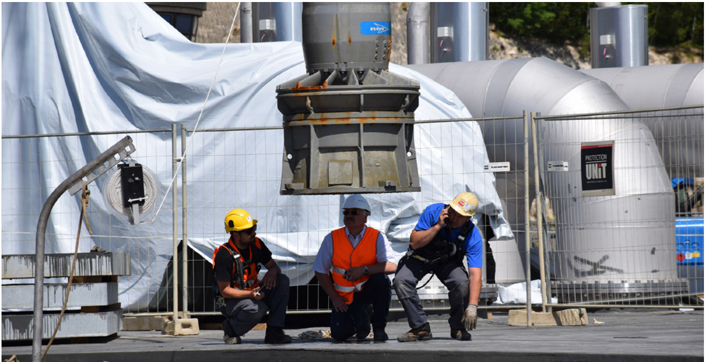
Careful working was required while placing the turbines
