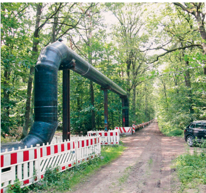
Figure 5: A bridge of steel pipes to maintain access to the forest
