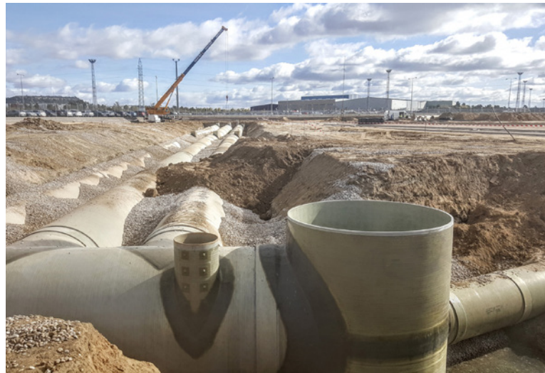
Figure 3: The GRP retention tank supplied for the FASA Renault Suppliers Park in the Spanish city of Valladolid holds 1,450 m 3
